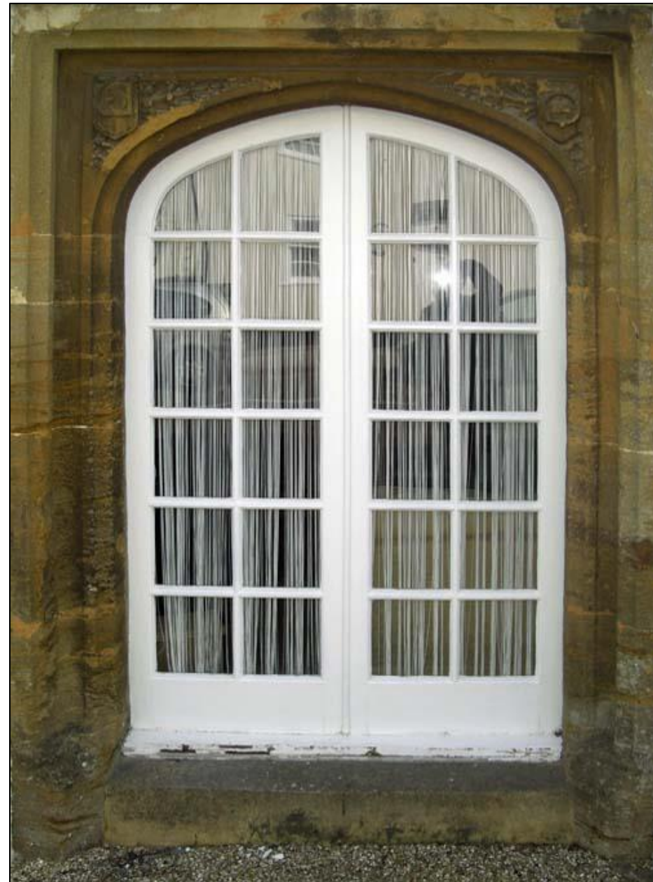
The doorway today after recent restoration
