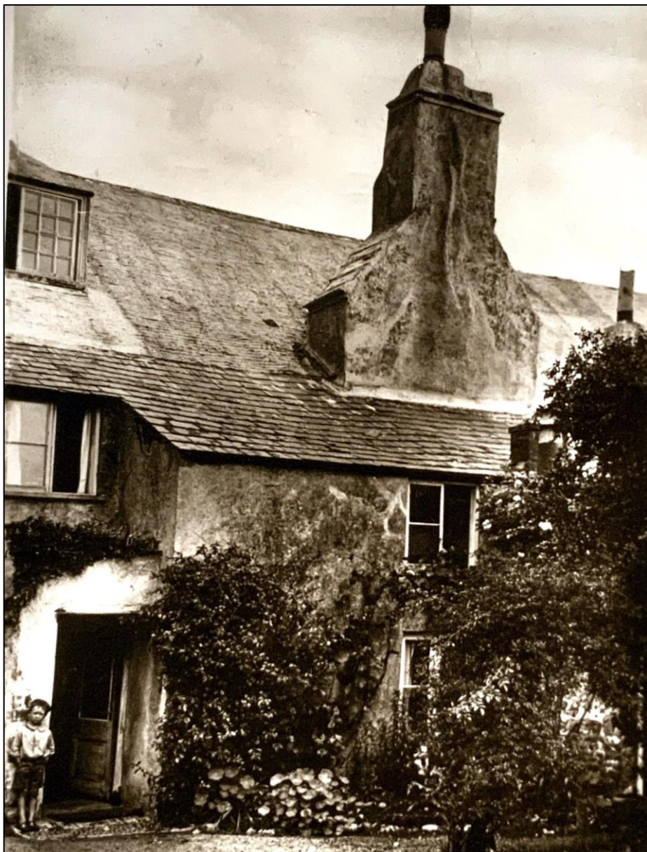
The massive chimney Stack in 1920 at the rear of the house.
